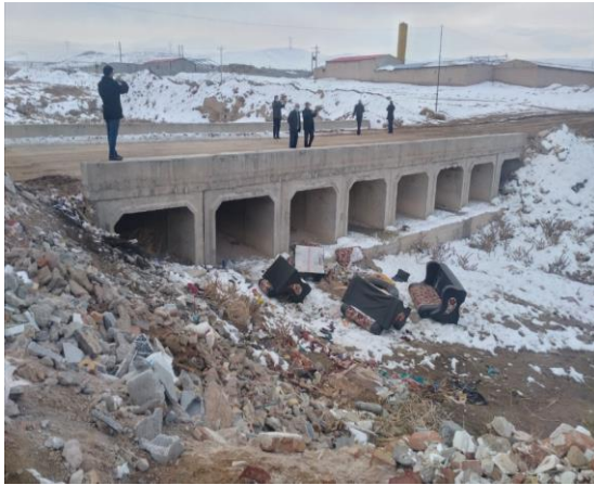
An example of obstacle in a surface- 3. Fig waterway in Tabriz city
